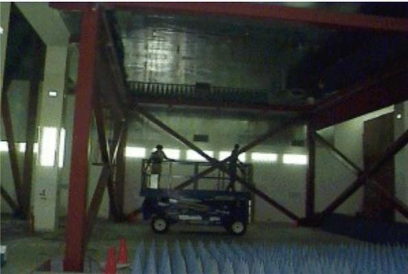
**Figure 12. Range #2, Support Frame Absorber Installation**
